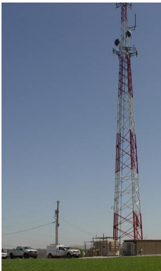
Motorola PTP 600 Series systems communicate from this KCP&L tower in Kansas City.
