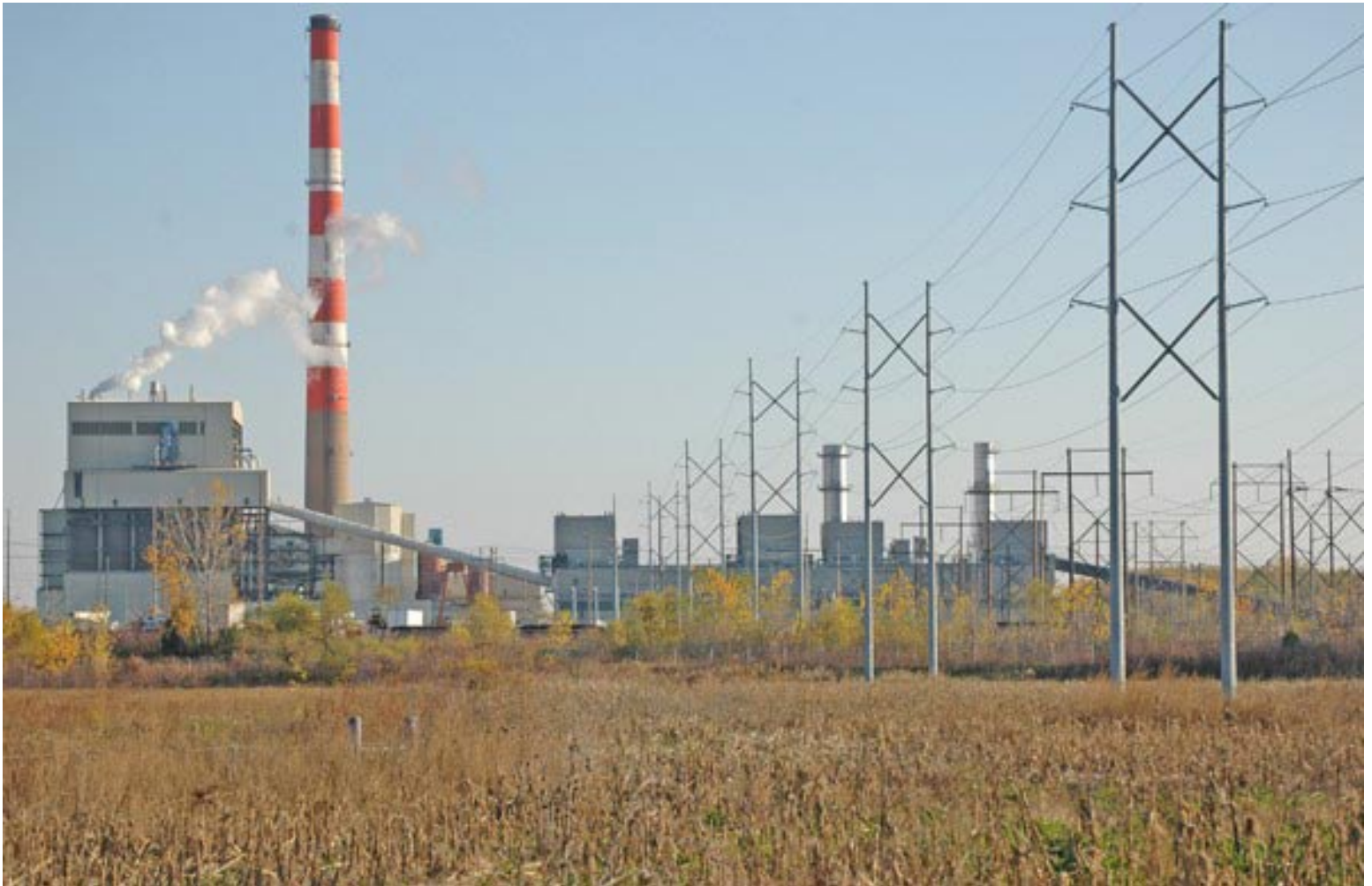
KCP&L's Hawthorn Station in Kansas City
